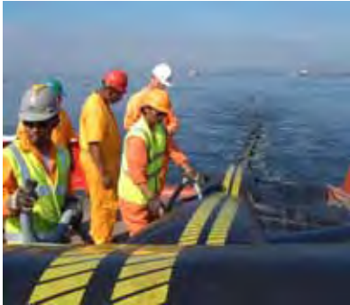
The first task is to contain the oil spill. This is done by using booms of various sizes. In the photograph above a RO-BOOM made of strong rubber is put in place. The RO-BOOMS can be up to 3.5 metres wide. However, small tasks on beaches, lakes and in harbours are handled with other more mobile versions of RO-BOOMS. Below an A-BOOM is carried to the scene of an accident by two men.
