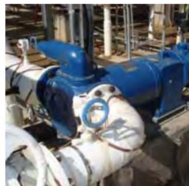
Magnet-driven Rotan ED pump for closed systems for toxic liquids
