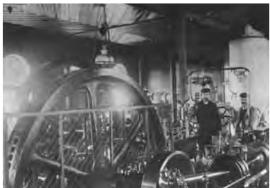
Steam driven pump for waterworks, 1895.
